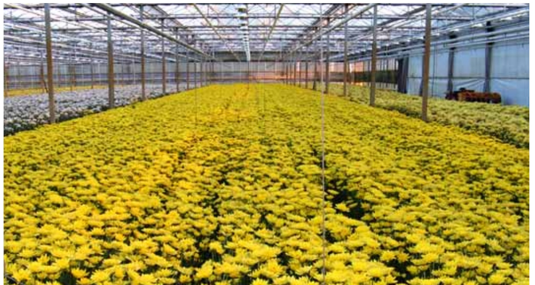
CHP greenhouse application
